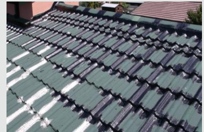
MORTAR IS REPLACE AND SEALED WITH HIGHBUILD S-200
