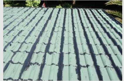
JOINS ARE SEALED WITH HIGHBUILD S-200
