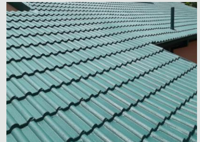
ROOF IS COATED WITH SEALROOF A-100
