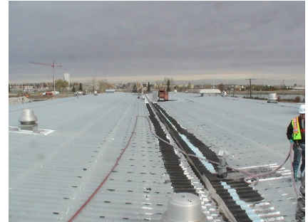
Prepping the roof
