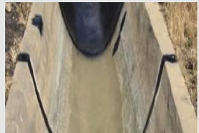
TROWELGRADE B-400 FOR JOINS AND CRACKS
